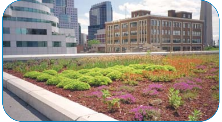
While reducing the urban heat island effect, a garden roof makes a significant contribution to the environment in delaying and reducing peak storm-water runoff.
