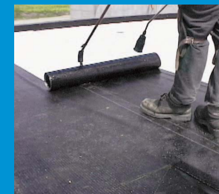
4 Weld cap sheet onto base sheet with torch (or with adhesive).
