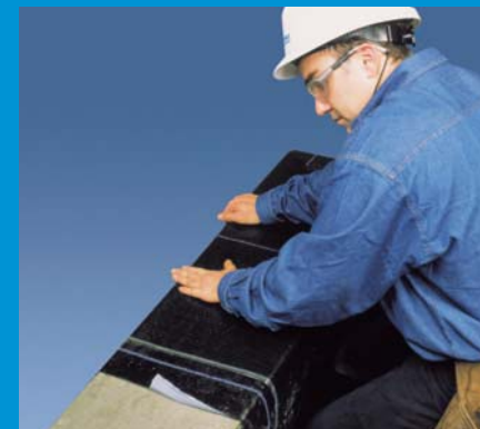
3 Install the base flashing membrane.
