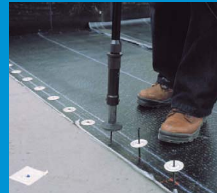
1 Install the base sheet dry and in parallel courses. Fasten the membrane in accordance with Soprema's technical manual.
