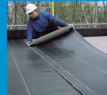
1 Install the base sheet dry and in parallel courses. Fasten the membrane in accordance with Soprema's technical manual.
